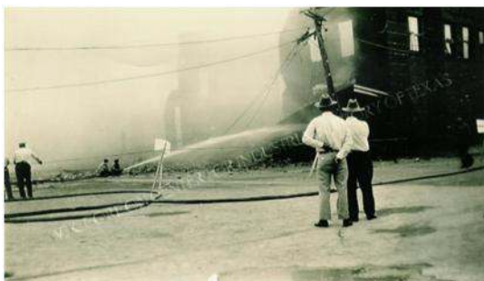
Fire destroys the market, hardware store, and general offices, September 14
